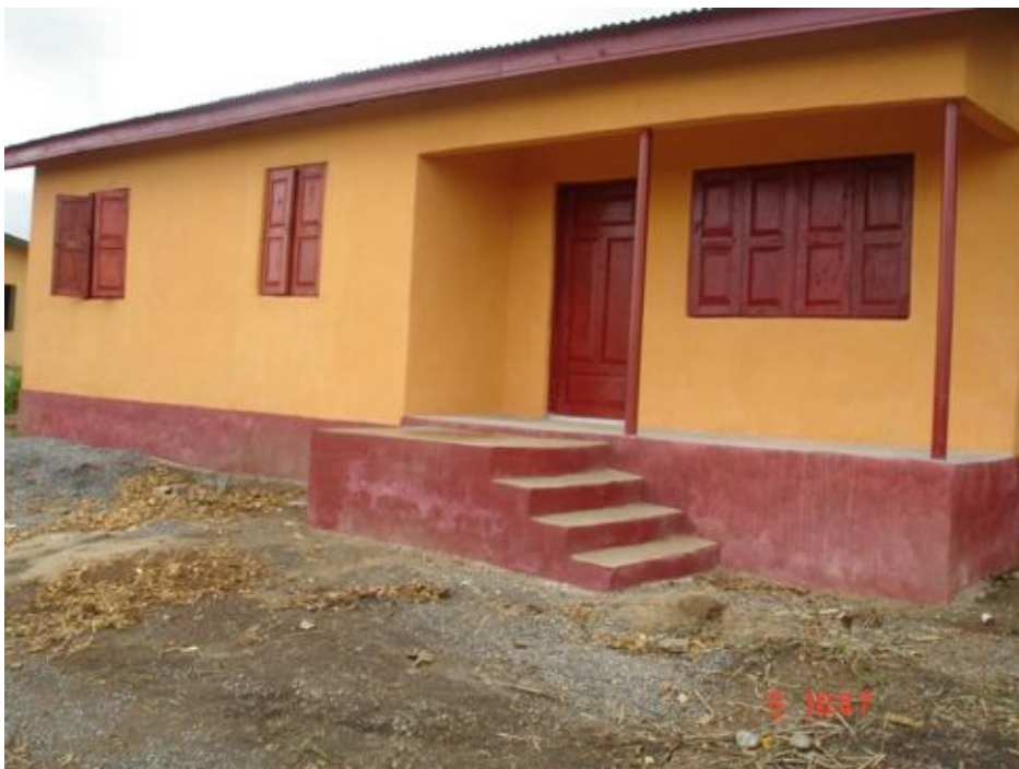
New Building C 71 Chapator Bah C/O Yorrer Jalloh 5 Bedrooms
