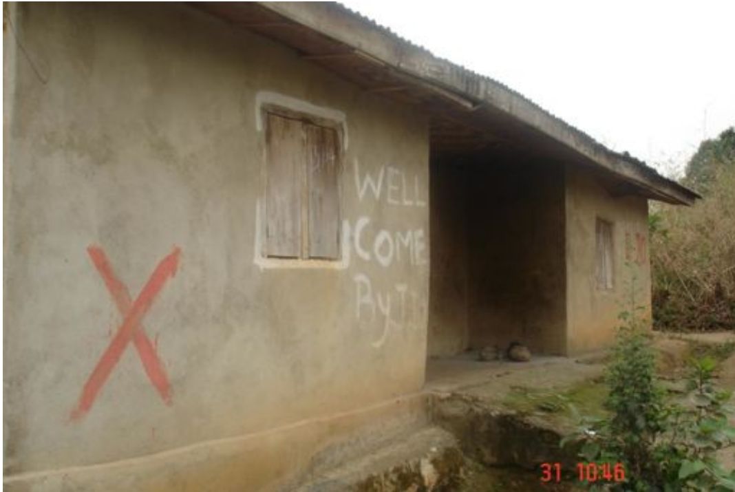
Old Structure Tamba Sam B 20 4 Bedrooms
