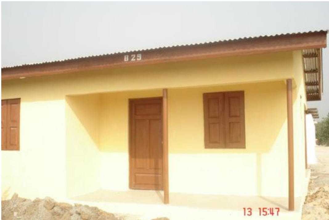
New Structure Sahr Denis Fengai B 29 3 Bedrooms
